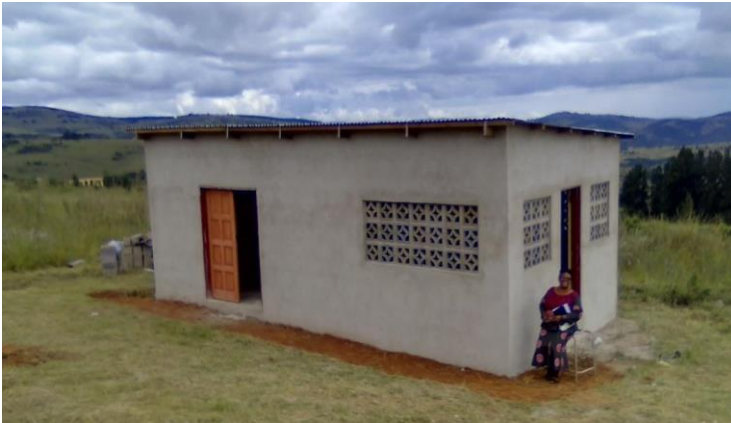
School Principal, Mrs Ncongwane stands proudly next to the completed poultry house.
