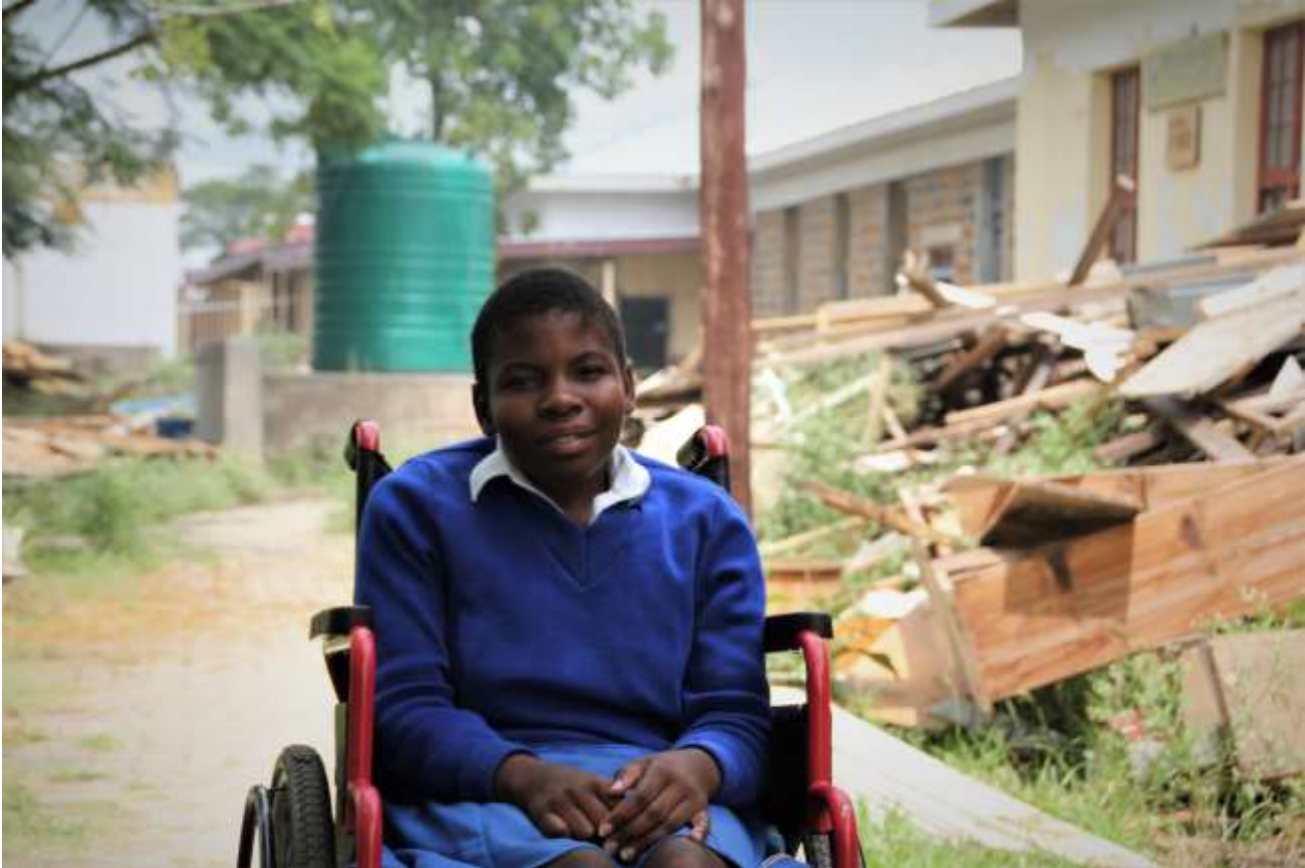
Sponsored student Siphesihle outside the Resource Centre for Deaf and partially-sighted children at St Joseph's School. Only the walls were left standing after the November storm.
