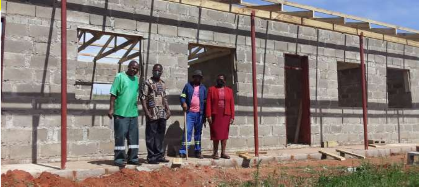
Classrooms for Forms 4 and 5 under construction at Nsingizini.
